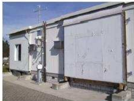
Figure 1a Outdoor test facility with removable façade element.
